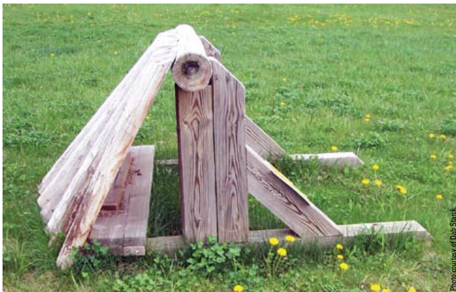
ABOVE: One way to stabilize jumps from tipping, says Starck, is to build a base that extends slightly past the back. NEXT PAGE: Stair step fences are some of the most "tippable" types of cross-country fences.
